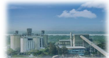
JSW Steel Ltd, Dolvi, Raigad; O&M of RMHS
