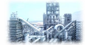
GCC, Integrated cement plant ~7,000 TPD and 33MWe WHR power plant
